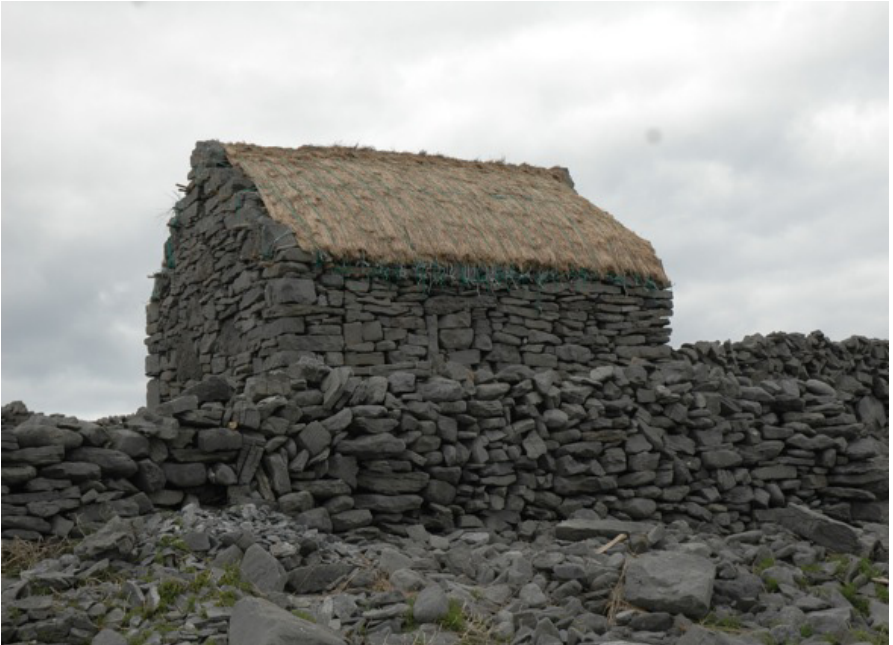
photo credit: Fidelma Mullane 'Seán Ó Conghaile' with a bundle of rye straw harvested on Inis Meáin; Inis Meáin field building for storing hay, recently thatched by Seán Ó Domhnaill with rye straw produced on the island
